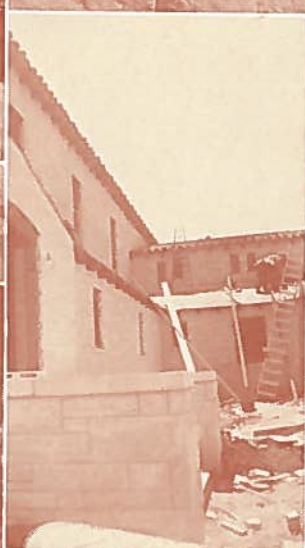
TILE ROOF BEING LAID July 5 TH
